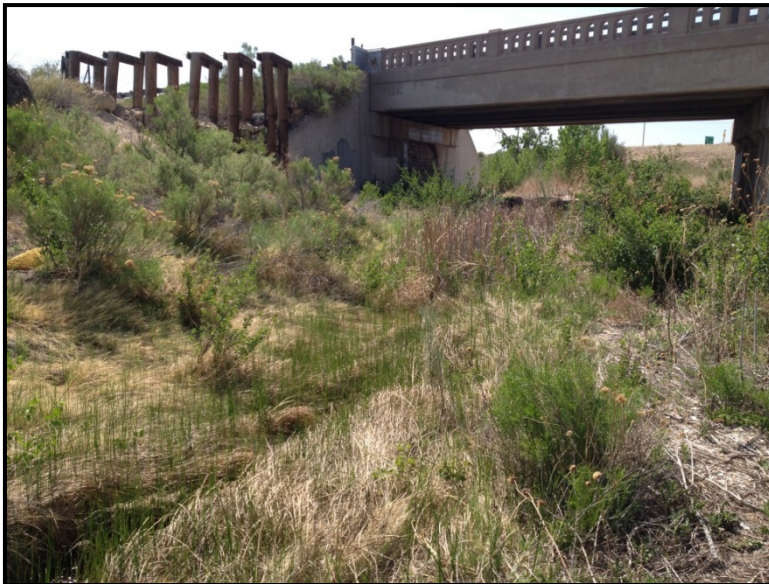
Photo 1 — Wetland WCN-1 in the background and Wetland WCS-1 in the foreground.
